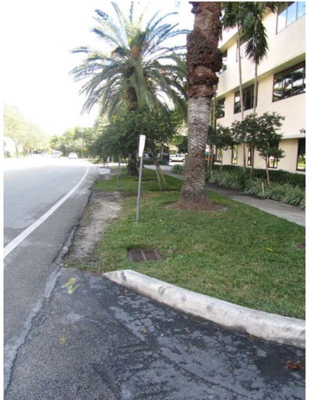
4. SIDEWALK. Once behind the hospital there is no continuous sidewalk. The path shown here is part of the ADA access into Doctor's Hospital.
