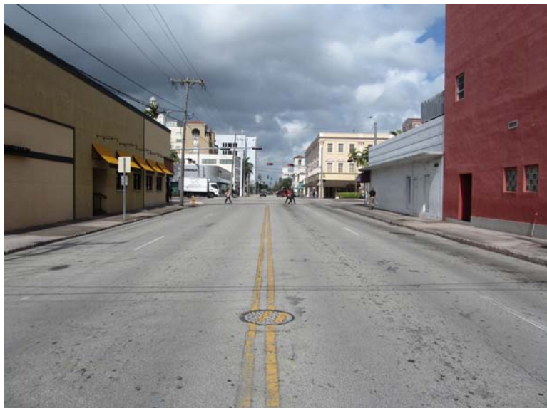
4. MAJOR INTERSECTION The intersection of Miracle Mile and Salzdeo is a pinch point for both automotive, bicycle, and pedestrian traffic. Use a center turn lane here to make room for on-street bike lanes.
