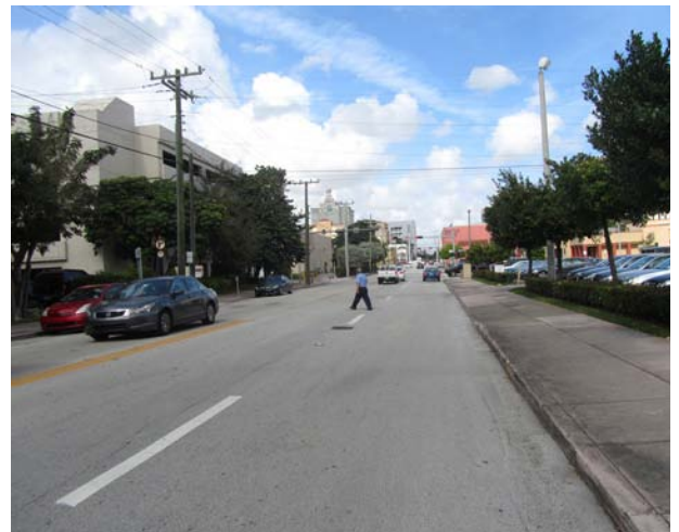
3. CROSSWALK Pedestrians frequently cross the street at mid-block locations due to poorly marked crosswalks.
