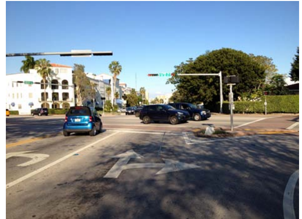
1. MAJOR INTERSECTION The intersection of University Drive and LeJeune Road is a pinch point for both automotive and pedestrian traffic. This right turn movement is a danger for cyclists. The approach and connection across LeJeune must be seamless and clear for bicyclists and motorists.
