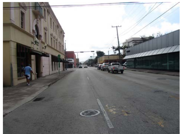
5. PINCH POINT. This section of Salzdeo is a pinch point for traffic traveling south, but not north. Use a center turn lane here to yield space for on-street bike lanes.
