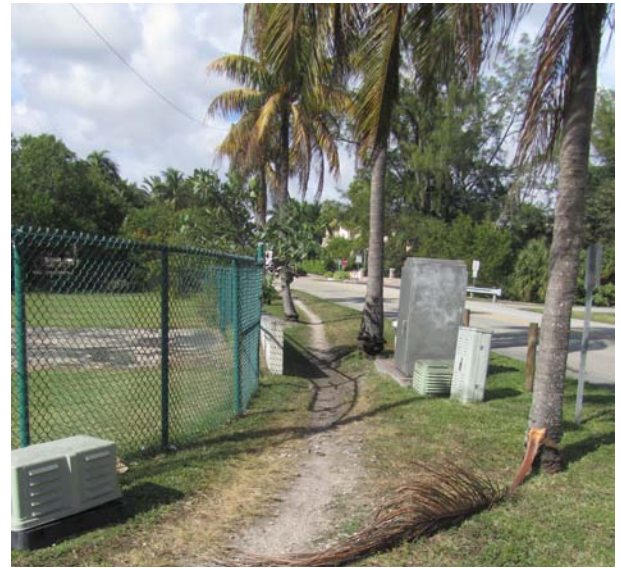
2. INTERSECTION A sidewalk is missing at the intersection of Carillo and Pisano Avenue.
