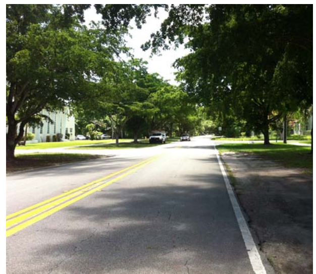
2. TYPICAL CONDITION Riviera is low speed and low volume - a perfect low street bicycle route.
