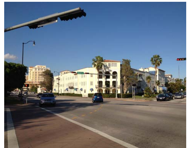
1. CROSSWALK This intersection has been the site of numerous pedestrian deaths over the years. The high speed nature of LeJeune is a challenge, as well as the wide right turn from LeJeune to University.
