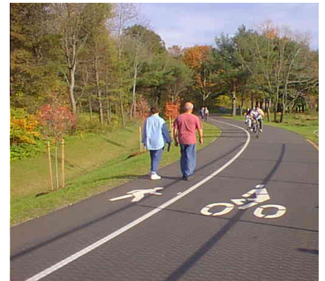
TYPICAL The typical shared-use path is 12' wide and can be paved with asphalt, concrete or higher quality pavers.
