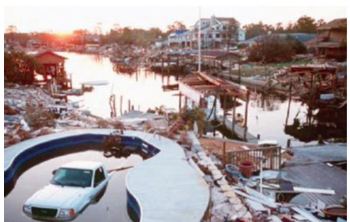
Figure 16: Damage after coastal storm.
