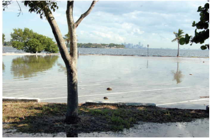
Figure 14: Flooding at Matheson Hammock from October 2010 high tide event.
